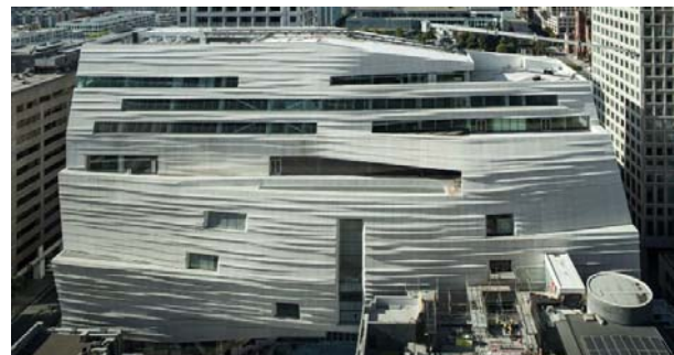
Figure 3: Cladding made from FRP composites
